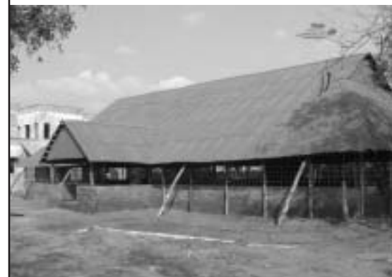
Temporary Chennai Yoga Hall
